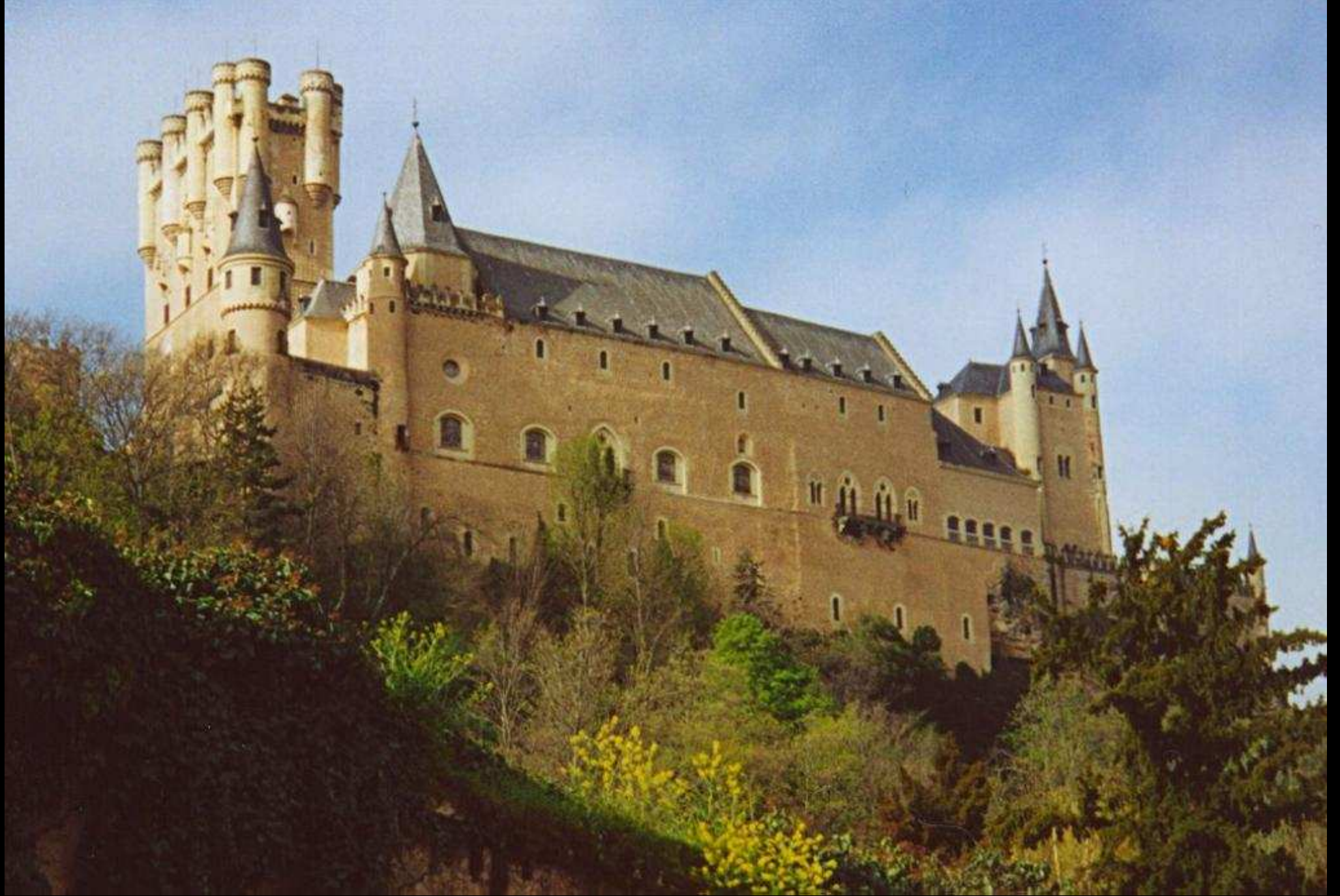
The Alcazar of Segovia, Spain. The military archive lowest range of small windows.
