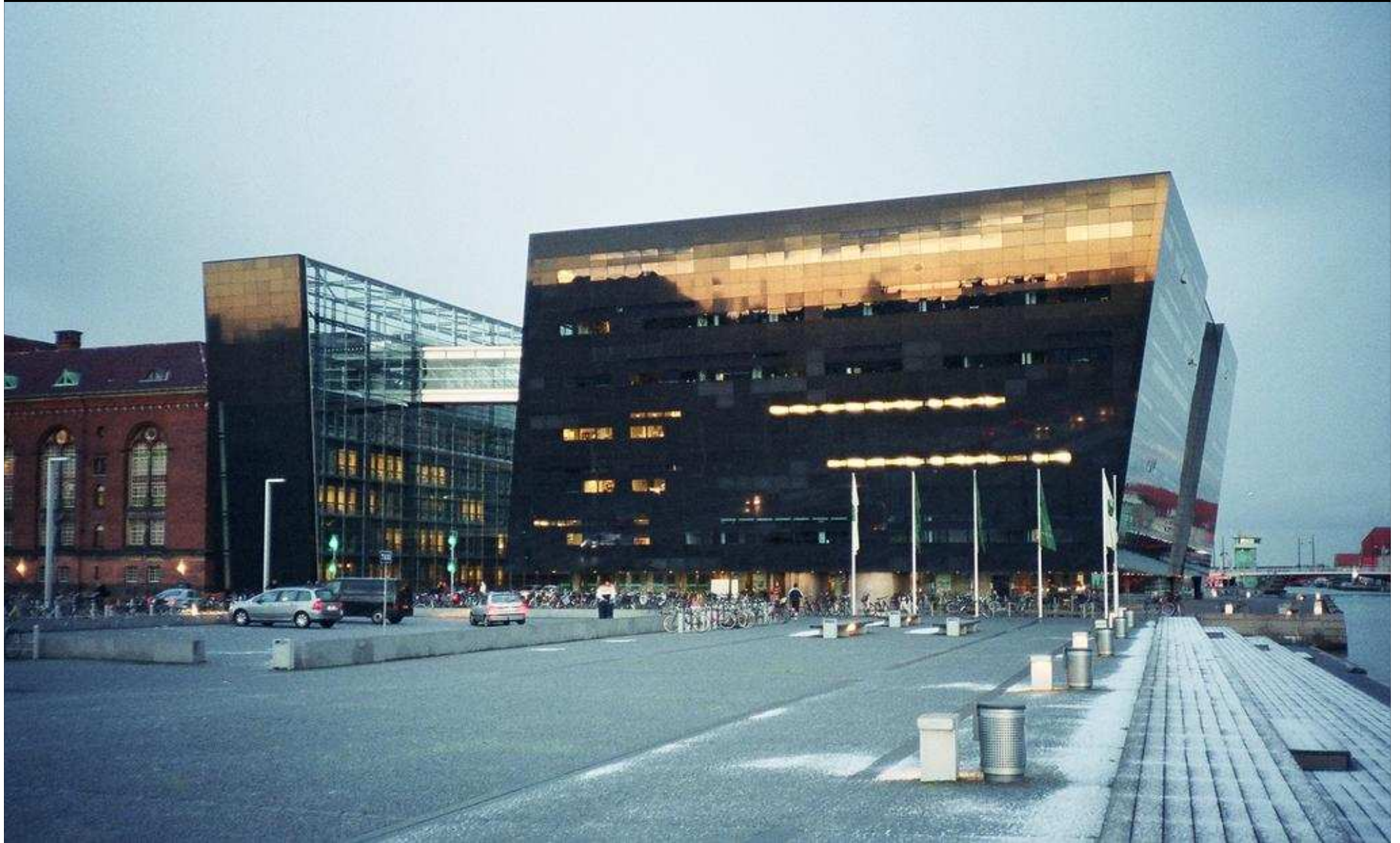
The Royal Library, Copenhagen. 1999. Architects Schmidt, Hammer and Lassen. The facade is black granite from Zimbabwe. An outward tilted wall cannot safely have high thermal capacity.
