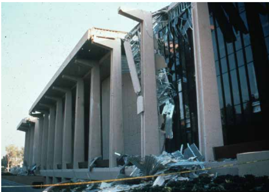
Figure 1 Exterior damage sustained by the Oviatt Library during the Northridge earthquake in 1994. Oviatt Digital Archives.
