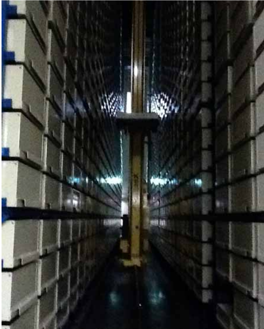
Figure 3. AS/RS rack structure.
