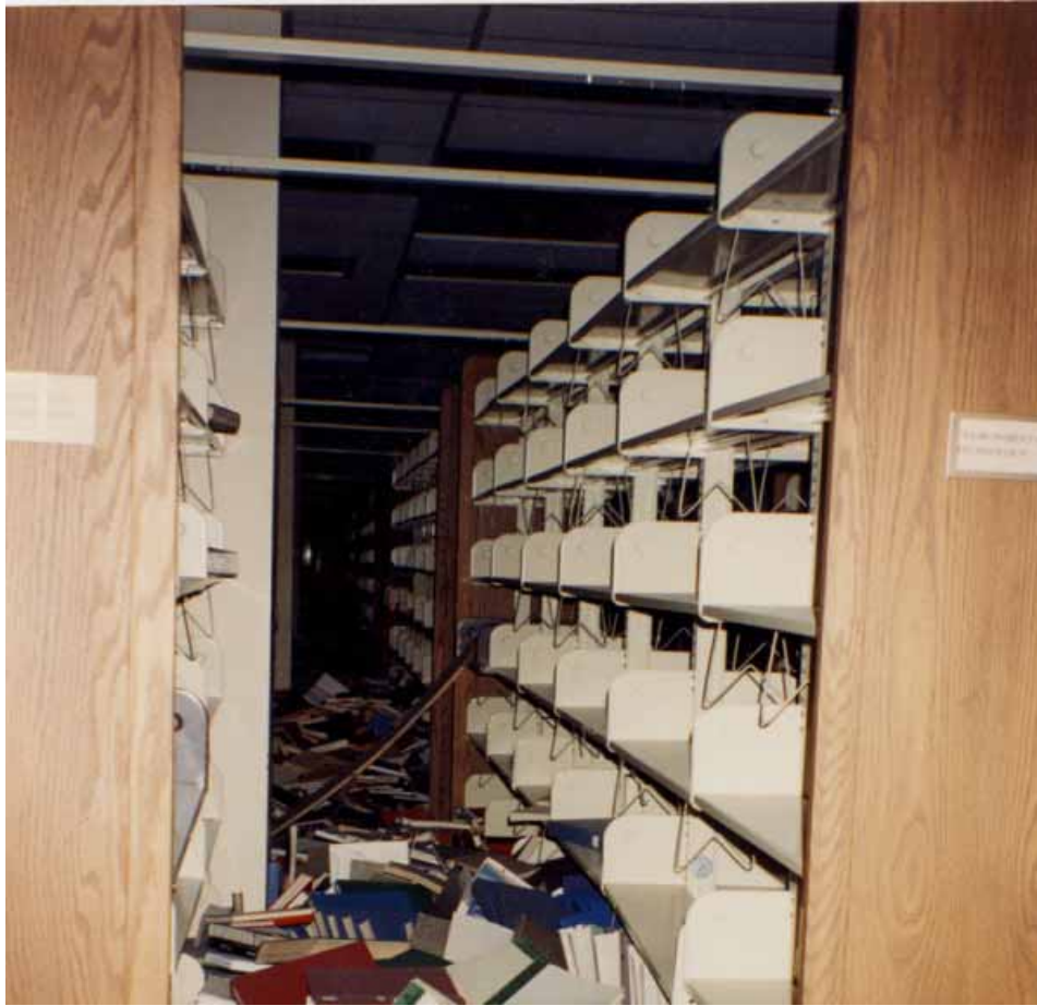
Figure 2 Damage to the stacks sustained by the Oviatt Library during the Northridge earthquake in 1994. Oviatt Digital Archives.
